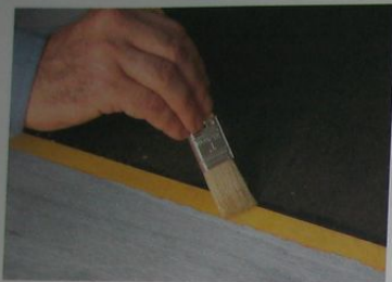
5. After the air bubbles are brushed out, use the first paste brush to carefully apply another layer of paste to the exposed margin of the backing paper (this is showing beyond the edges of the good paper).
